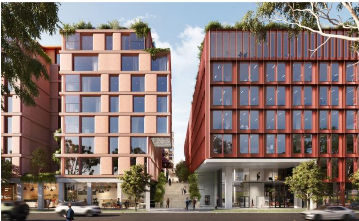
Figure 13: Photomontage of the BVN winning scheme (part of the Wattle Street elevation)
