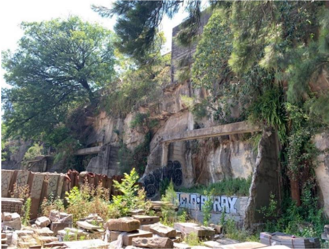
Figure 2: Cliff face along the site's eastern boundary adjoining Jones Street
